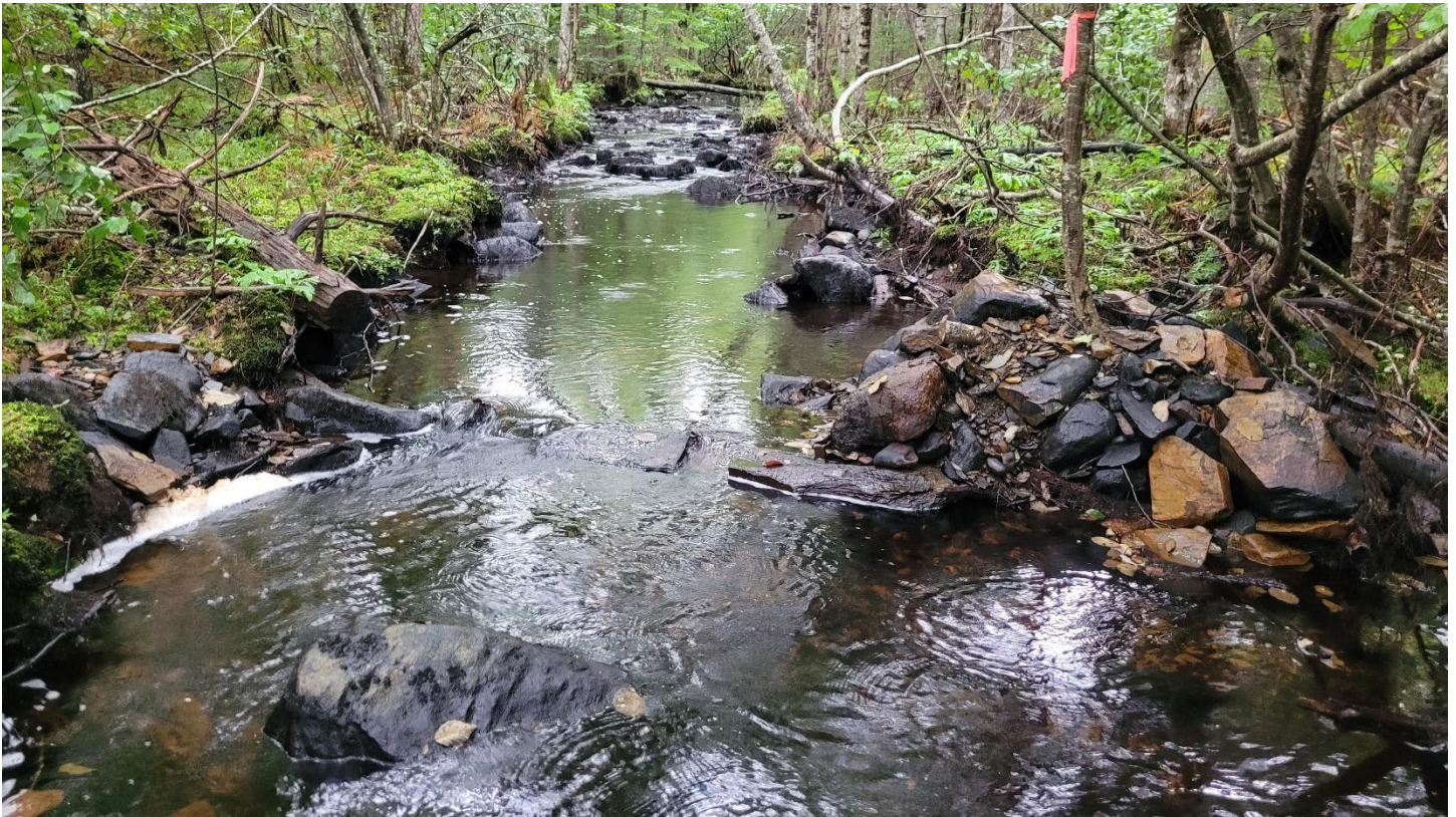
Site 11 – Rock sill 11 with deflector - before (above) and after (below)
