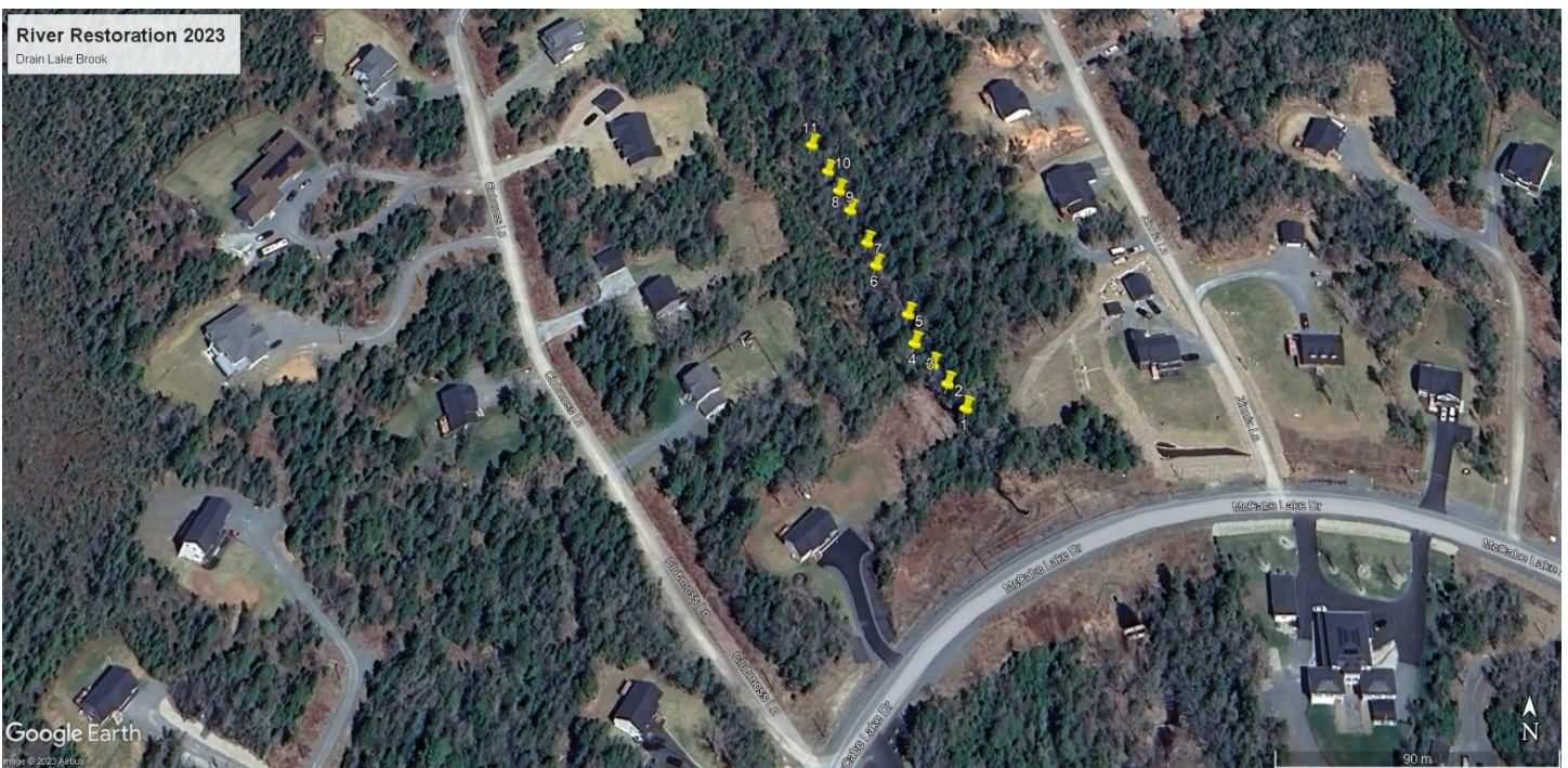
River Restoration 2023 – Drain Lake Brook habitat restoration installations (sites 1 through 11 – one rock sill and one deflector installation at each site).
